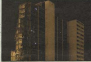
Cabrini-Green is torn down
